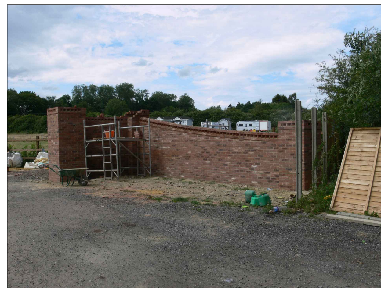
NOTE 3 - ENTRANCE WING WALLS
